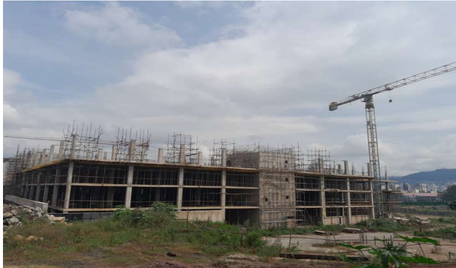
Figure 9: Progress of the construction of the Advanced Multi-Specialty Hospital
